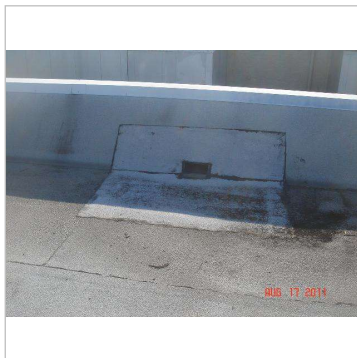
Figure 19B - repair at scupper drain
