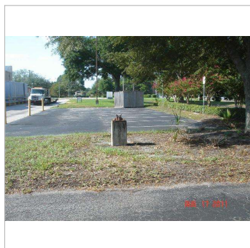
Figure 1A - Public street lamp missing
