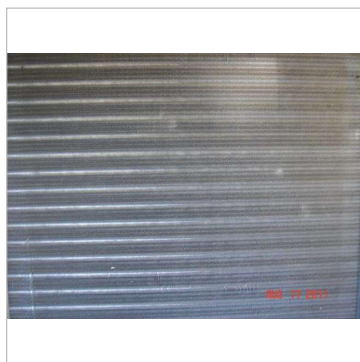
Figure 14A - Evaporator coil
