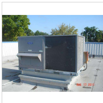
Figure 12A - Carrier roof top packaged system
