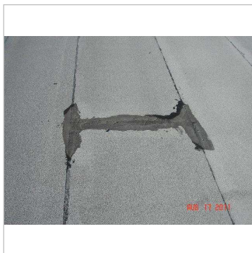
Figure 5B - patched seam at overlap
