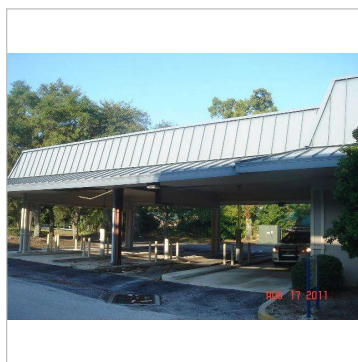
Figure 7A - metal standing seam overhang and fascade
