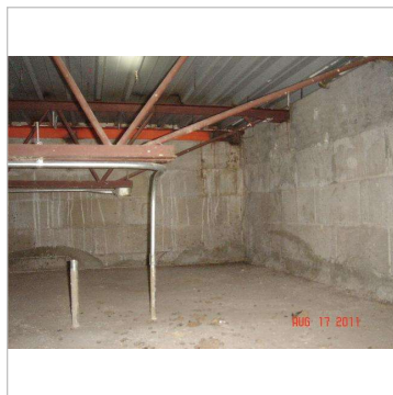
Figure 3A - View of steel truss supporting metal roof deck
