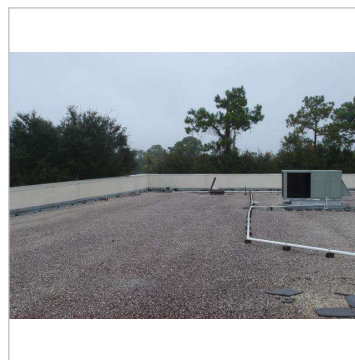
Figure 10C - gravel built up roof-2
