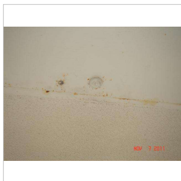
Figure 16A - access hatch to facade is painted over
