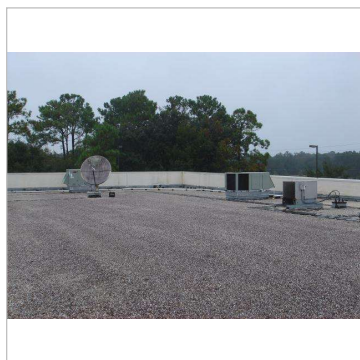
Figure 10A - gravel built up roof
