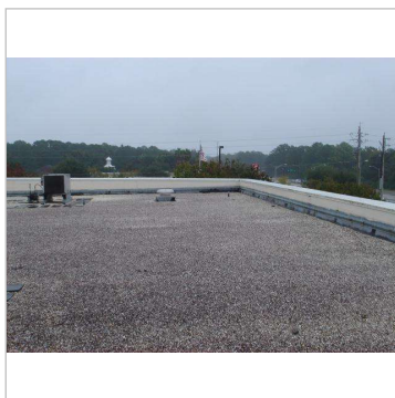
Figure 10B - gravel built up roof-3
