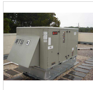
Figure 21C - rtu-3 6ton
