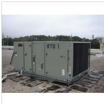
Figure 21A - Rtu-1 15 ton
