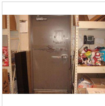
Figure 8B - rear entry to store room
