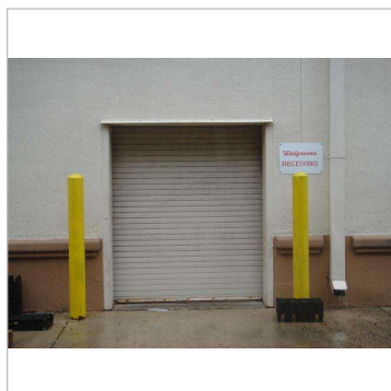
Figure 24A - loading or receiving dock
