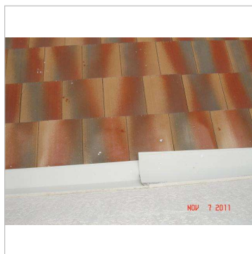
Figure 14A - tile roof
