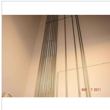
Figure 18A - extruded metal conduit
